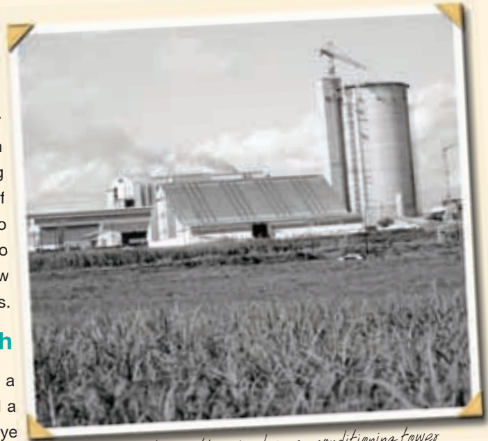
ubombo factory with refined sugar conditioning tower under construction
