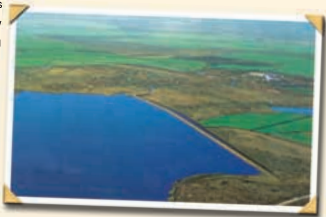
Van Eck dam, Ubombo's main water supply
