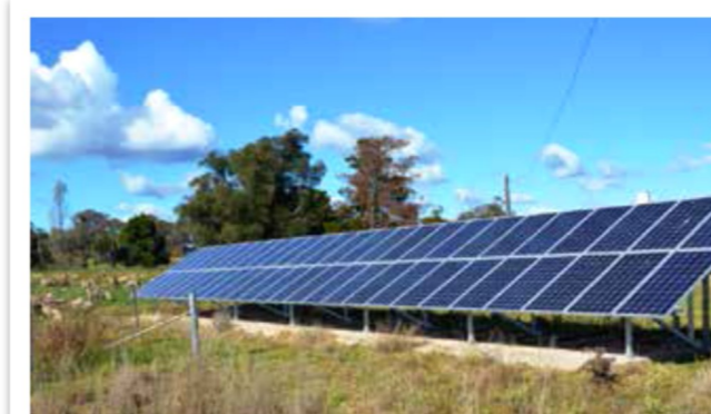
Figure 1: Typical solar panels used in irrigation
