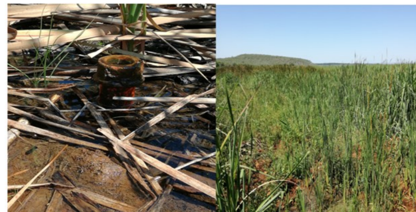
Figure 5: Leaking riser which has resulted in serious waterlogging
